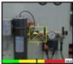
FACE A SMALL LEAK
